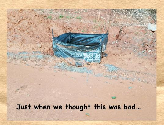
They build a berm in the road to direct all the silt and water to a compromised storm drain that goes directly to "Red Lake" without a single prophylactic measure to slow or stop the silt path to the lake.
